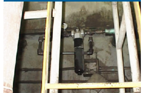
RLT filter on an ID fan.
